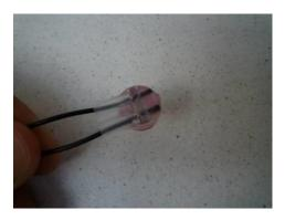
Insert the trimmed wire ends into the Scotchlok $^{\text{\tiny M}}$  connector. Do not strip the wires. Make sure all wires are inserted fully to the end of the tunnels, past the metal connector element.
